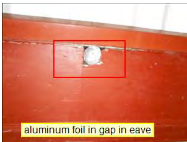
2.5 Item 3(Picture) Eave on back of home
