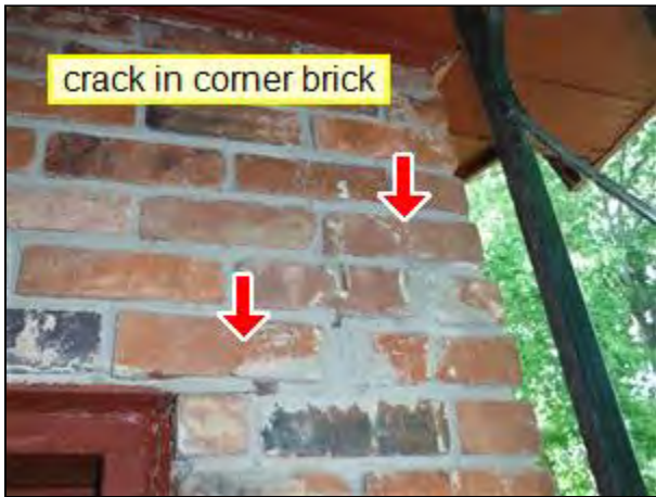
2.0 Item 9(Picture) Back corner of home
