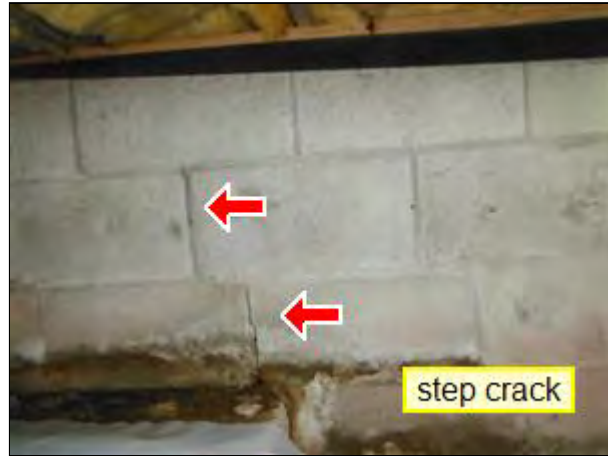
5.1 Item 2(Picture) Crawspace walls
