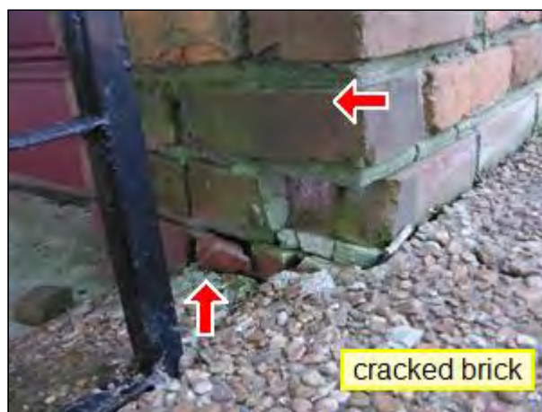
2.0 Item 10(Picture) Back right corner
