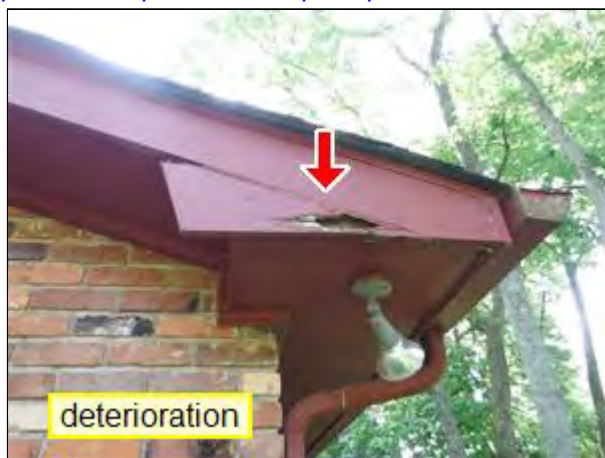
2.5 Item 1(Picture) Eave on corner
