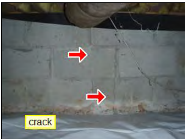
5.1 Item 5(Picture) Crawspac walls
