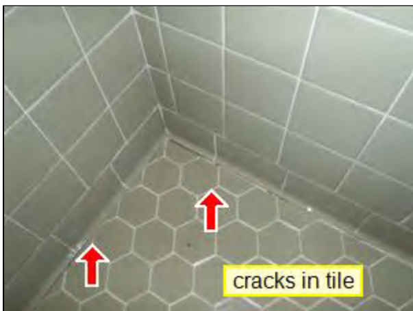
6.1 Item 3(Picture) Upstairs Shower Floor
