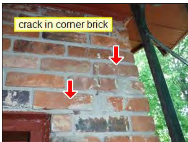
2.0 Item 9(Picture) Back corner of home
