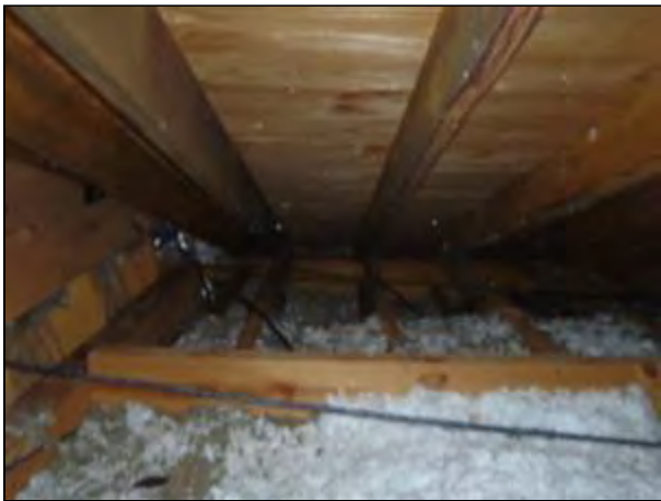
5.5 Item 9(Picture) Attic
