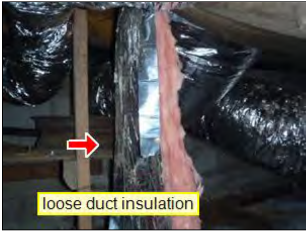
8.3 Item 1(Picture) Duct in crawlspace
