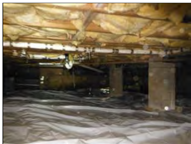
5.0 Item 1(Picture) Crawlspace
