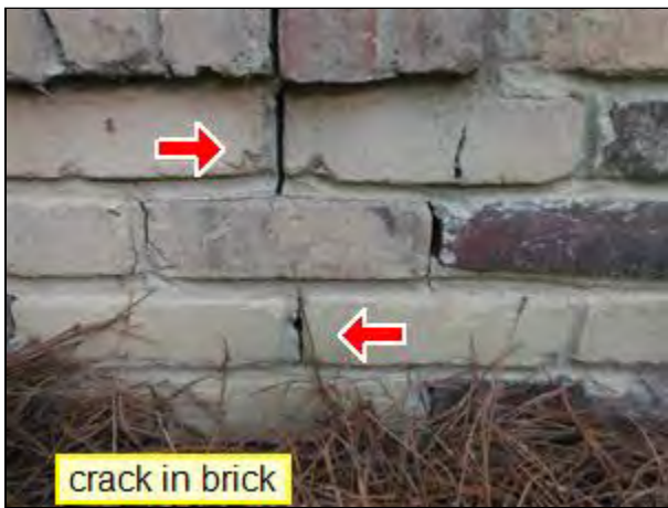
2.0 Item 3(Picture) Brick Exterior
