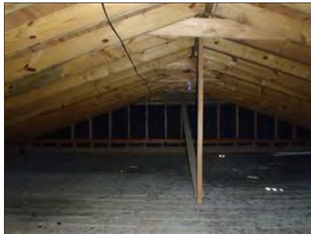
5.5 Item 6(Picture) Roof structure
