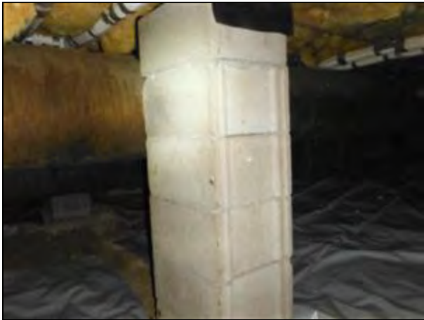
5.2 Item 1(Picture) Concrete Piers
