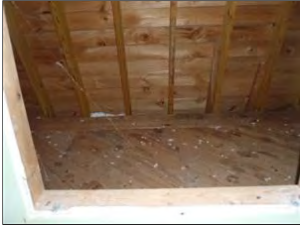
5.5 Item 1(Picture) Roof structure
