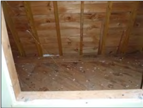
5.5 Item 1(Picture) Roof structure
