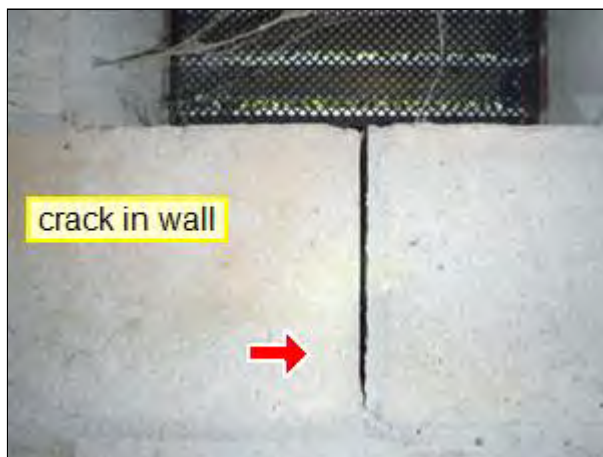
5.1 Item 3(Picture) Crawspace wall
