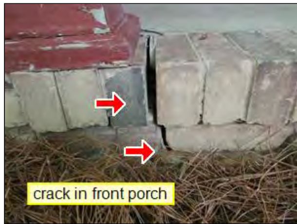
2.0 Item 4(Picture) Front porch
