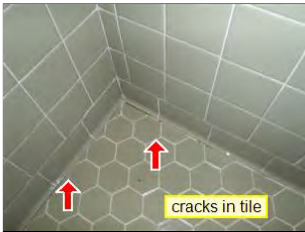
6.1 Item 3(Picture) Upstairs Shower Floor
