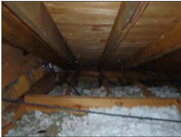
5.5 Item 9(Picture) Attic
