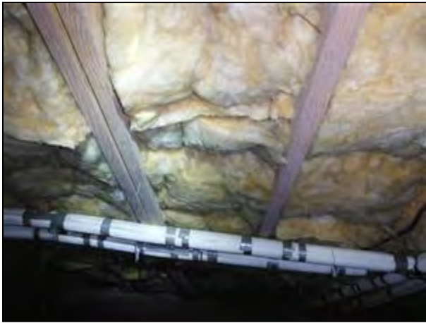
9.1 Item 1(Picture) Insulation in sub floors
