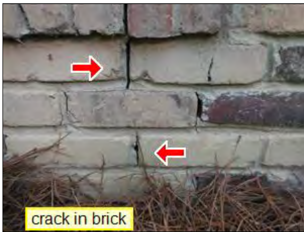
2.0 Item 3(Picture) Brick Exterior
