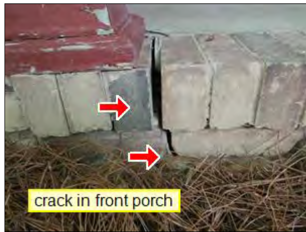
2.0 Item 4(Picture) Front porch
