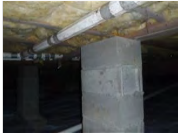
5.2 Item 2(Picture) Concrete Piers
