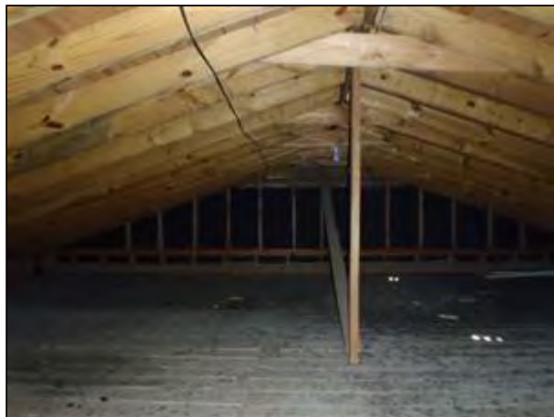
5.5 Item 6(Picture) Roof structure
