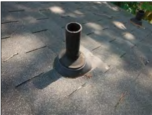
1.2 Item 3(Picture) Plumbing vent boots
