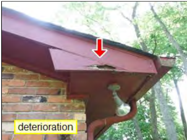
2.5 Item 1(Picture) Eave on corner
