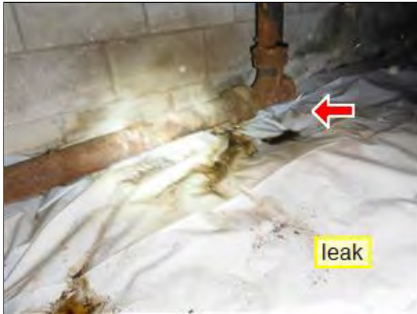
6.0 Item 1(Picture) Plumbing drain under hall toilet
