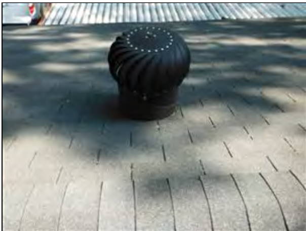
9.3 Item 1(Picture) Attic Vents
