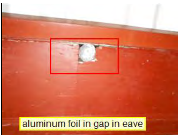
2.5 Item 3(Picture) Eave on back of home
