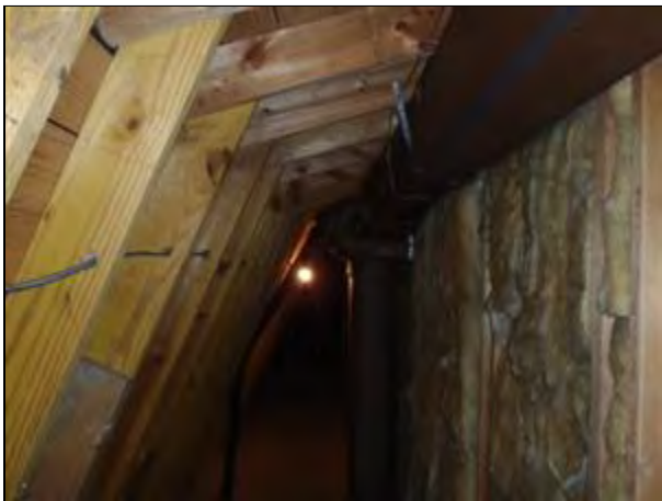
5.5 Item 5(Picture) Roof structure
