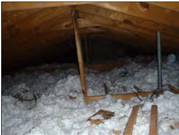
9.0 Item 1(Picture) Attic Insulation
