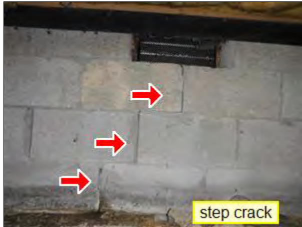
5.1 Item 1(Picture) Crawspace wall
