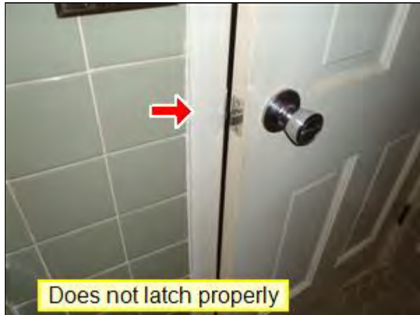
4.5 Item 1(Picture) Upstairs Bathroom Door
