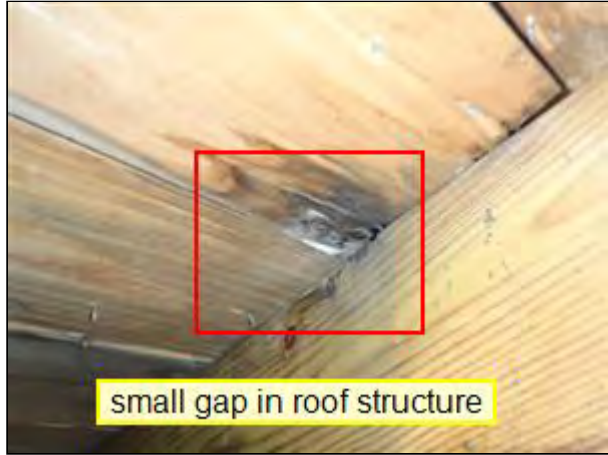
5.5 Item 8(Picture) Roof over garage area
