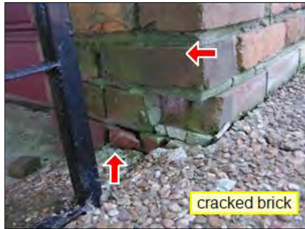
2.0 Item 10(Picture) Back right corner
