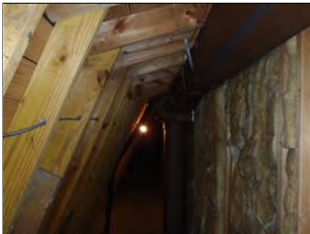
5.5 Item 5(Picture) Roof structure
