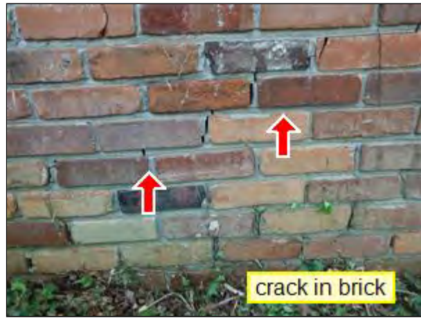
2.0 Item 2(Picture) Brick Exterior
