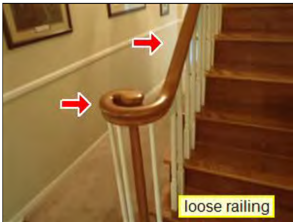
4.3 Item 1(Picture) Railing
