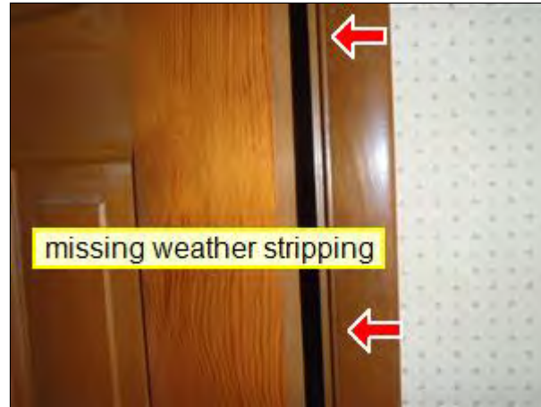
4.5 Item 2(Picture) Door to attic
