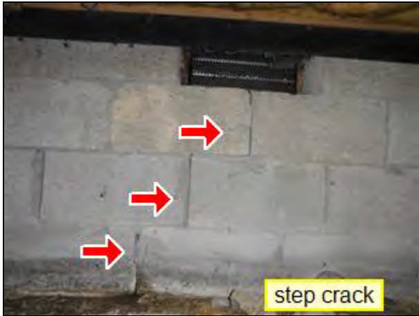
5.1 Item 1(Picture) Crawspace wall
