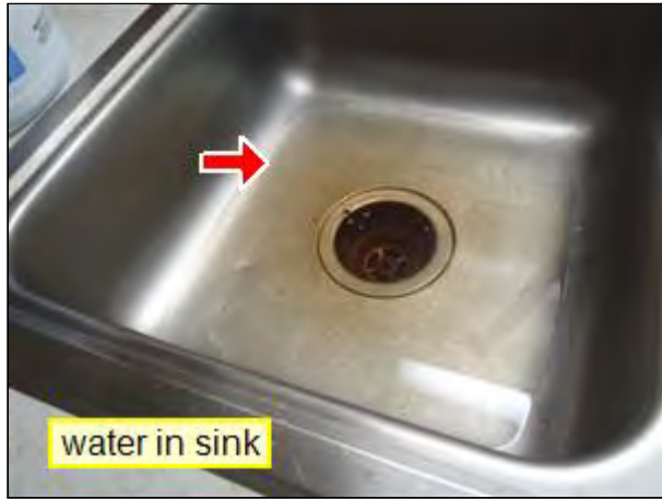
6.1 Item 2(Picture) Kitchen sink
