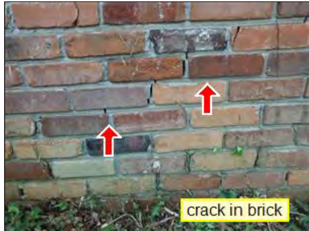
2.0 Item 2(Picture) Brick Exterior
