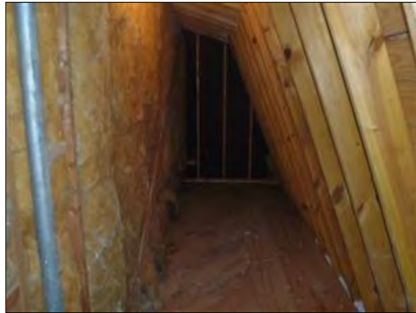
5.5 Item 2(Picture) Attic
