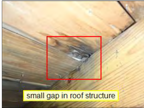
5.5 Item 8(Picture) Roof over garage area
