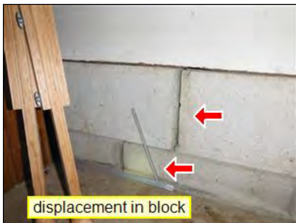
3.1 Item 1(Picture) Garage front wall
