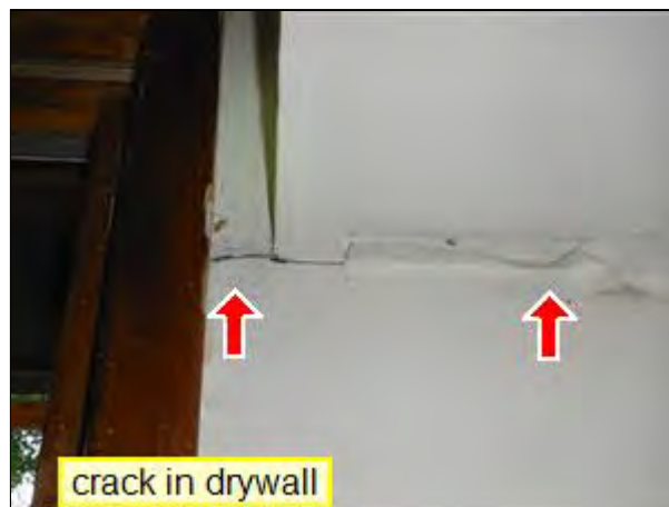
3.1 Item 2(Picture) Garage
