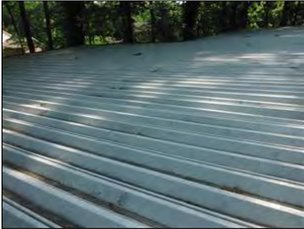
1.0 Item 1(Picture) Carport Roof
