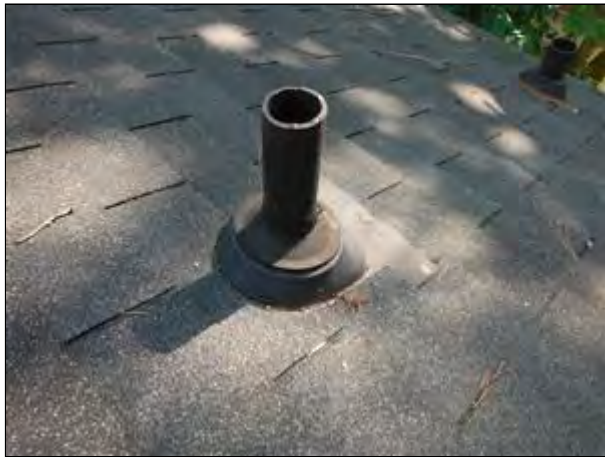
1.2 Item 3(Picture) Plumbing vent boots
