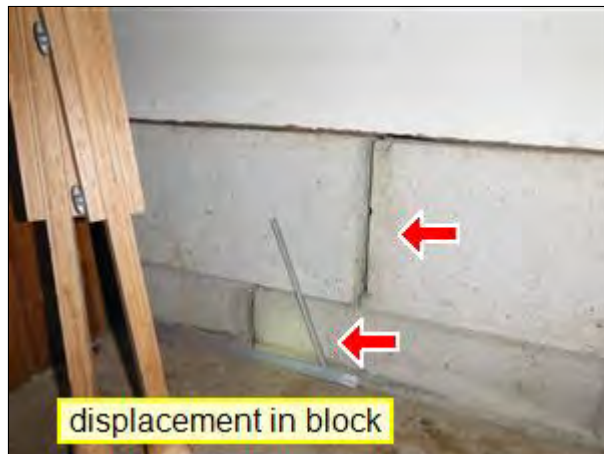
3.1 Item 1(Picture) Garage front wall
