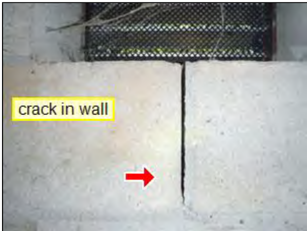
5.1 Item 3(Picture) Crawspace wall
