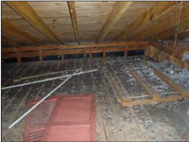
5.5 Item 7(Picture) Roof structure
