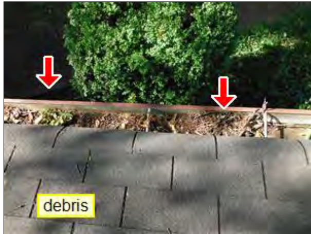
1.3 Item 1(Picture) Gutters
