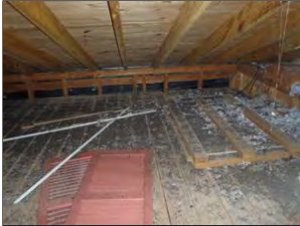
5.5 Item 7(Picture) Roof structure
