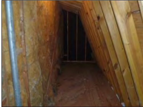
5.5 Item 2(Picture) Attic
