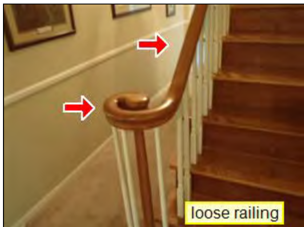
4.3 Item 1(Picture) Railing
