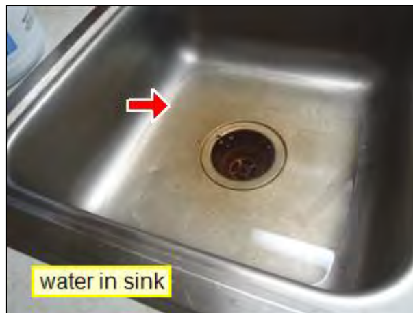
6.1 Item 2(Picture) Kitchen sink
