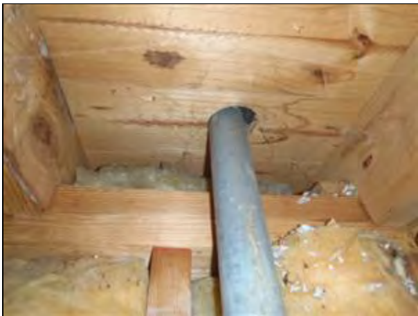
5.5 Item 3(Picture) Roof structure
