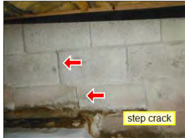
5.1 Item 2(Picture) Crawspace walls
