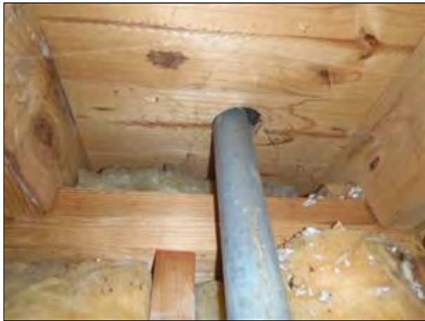
5.5 Item 3(Picture) Roof structure
