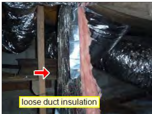
8.3 Item 1(Picture) Duct in crawlspace
