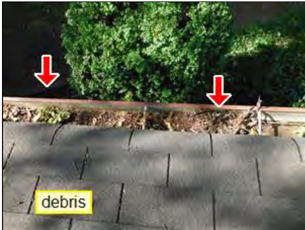
1.3 Item 1(Picture) Gutters
