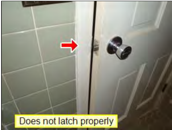
4.5 Item 1(Picture) Upstairs Bathroom Door
