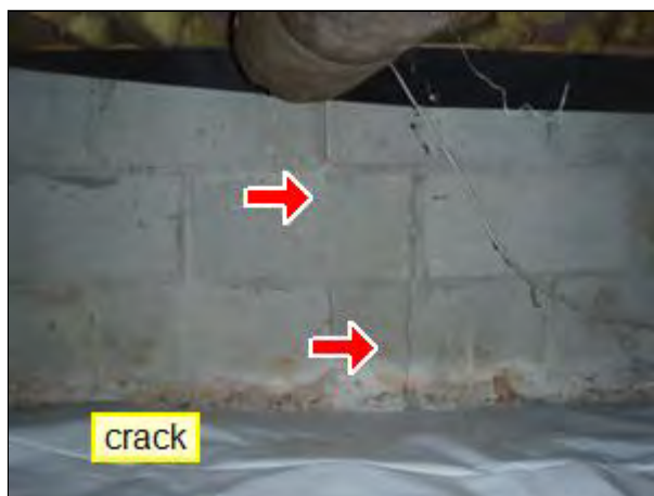
5.1 Item 5(Picture) Crawspac walls
