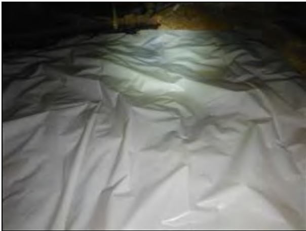
9.2 Item 1(Picture) Vapor Barrier
